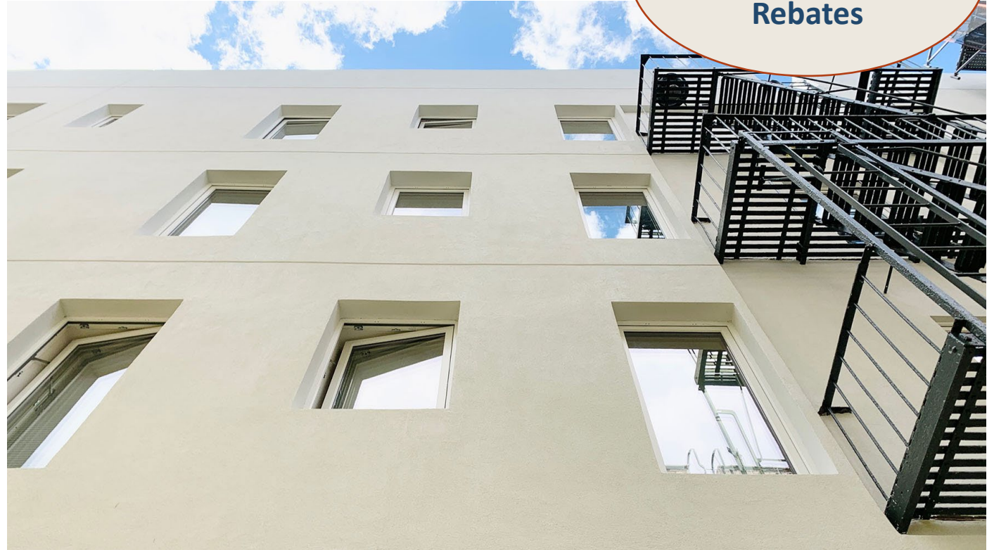
Riseboro, Brooklyn, Passive House, 80% energy reduction
